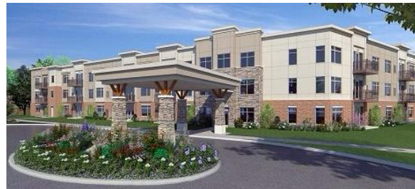
December 23, 2016: WHEFA closed bonds for Evergreen Retirement Community's construction and equipping of a new 109,000 square-foot, three-story addition on the north side of the Evergreen campus in Oshkosh, Wisconsin, to contain up to 62 new independent living units. The project will also include the relocation of the campus main entrance, additional parking, a new library and more common spaces.
